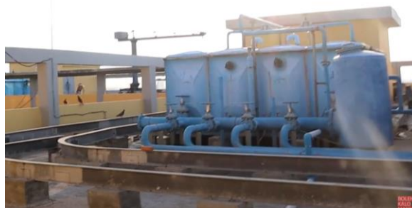
Figure 3.9. The roof finish is only gray concrete
