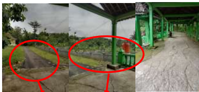
The expansion, construction of boundary walls, and installation of a water tank were carried out using contributions from the residents of Banyusri Village.
