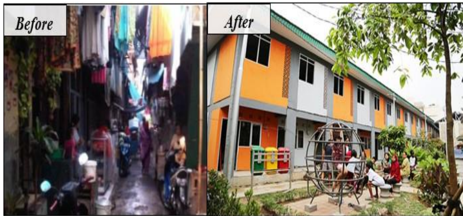
Figure 8. Before and After Condition in KDP Petogogan Village (Source: DPGP DKI Jakarta, 2013c)
