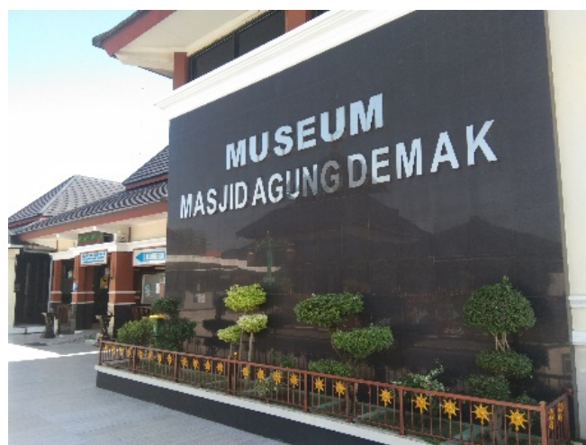
Figure 1. Demak Grand Mosque Museum building that has been build since 2011.
